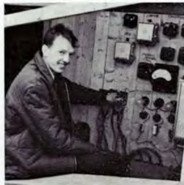
Electrician G. E. Davies at work on the switchboard in the main marquee
