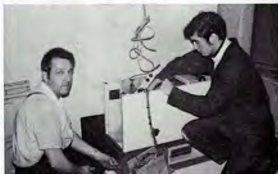
William Hargreaves (contracting electrician) and apprentice David Gambon, at work installing one of the Electricaire units at Litherland
